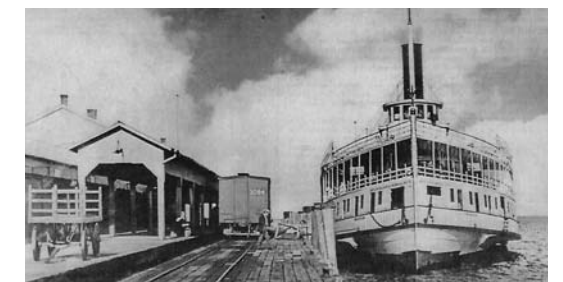
Train and steamboat at Love Point exchange passengers. Sidewheeler Westmorland with the train waiting alongside at Love Point
