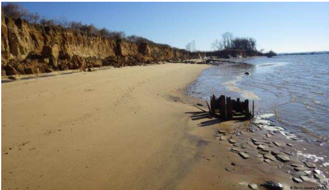
Figure 3.28. The image shows the collapsed well feature on December 23rd, 2018.
