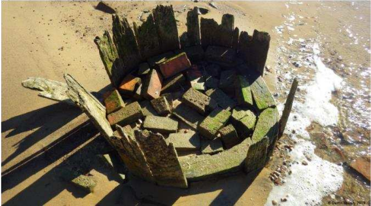
Figure 3.29. The image shows the bottom portion of the well feature and how it was constructed. The wooden hogs head surrounded the brick shaft. At the bottom a series of hand-hewn wooden planks or timbers were installed to strengthen the well's foundation and possibly serve as a filtering devise.
