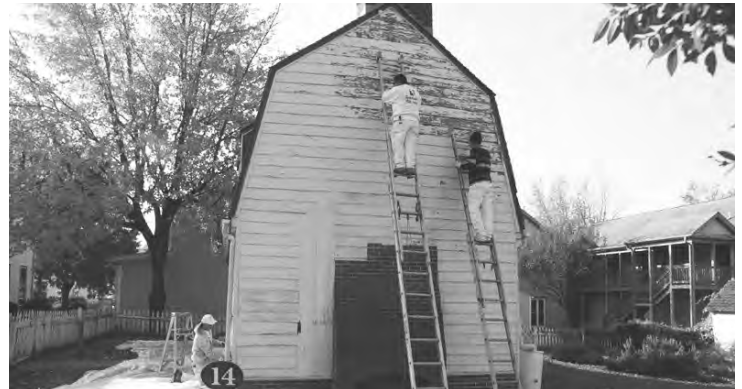
Chesapeake Property Finishes' workers scraping old paint and mold from the Cray House at top; below right, worker prepares surface for painting; at right, removing deteriorated siding for replacement; below, Lundberg Builder's carpenter Bill Rochow priming siding.
