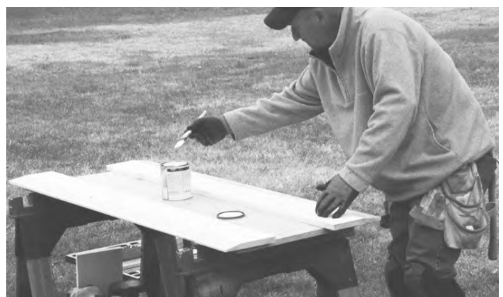
Chesapeake Property Finishes' workers scraping old paint and mold from the Cray House at top; below right, worker prepares surface for painting; at right, removing deteriorated siding for replacement; below, Lundberg Builder's carpenter Bill Rochow priming siding.
