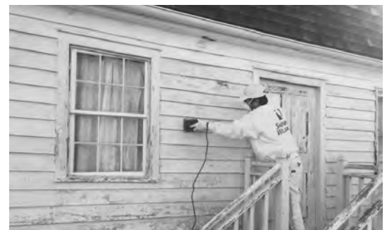
Chesapeake Property Finishes' workers scraping old paint and mold from the Cray House at top; below right, worker prepares surface for painting; at right, removing deteriorated siding for replacement; below, Lundberg Builder's carpenter Bill Rochow priming siding.
