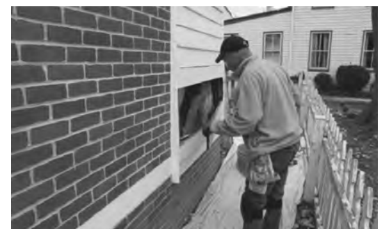
Chesapeake Property Finishes' workers scraping old paint and mold from the Cray House at top; below right, worker prepares surface for painting; at right, removing deteriorated siding for replacement; below, Lundberg Builder's carpenter Bill Rochow priming siding.
